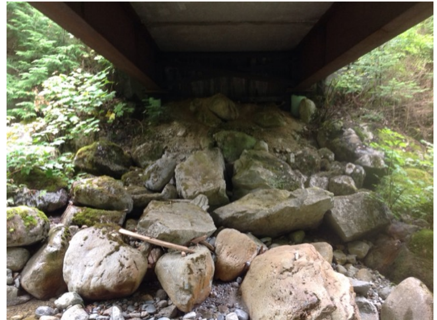
Left Bank Abutment when facing downstream
