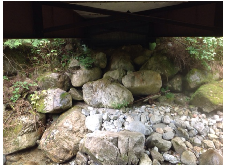
Right Bank Abutment when facing downstream
